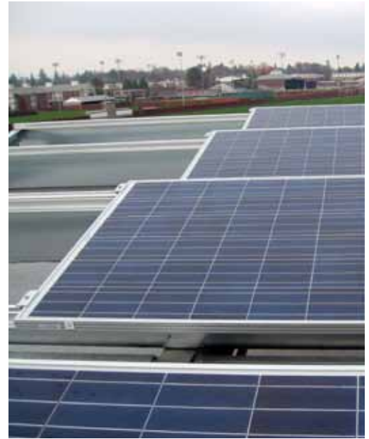
Ninety-six solar panels sit on top of the building, providing over three percent of the building's energy use.
