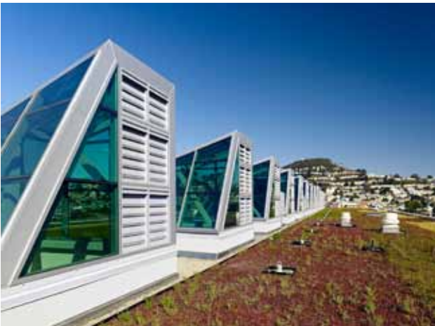
(Above) Interior ventilation louvers rather than traditional ductwork are a source of air conditioning. (Right) Advanced engineering tools were employed by Interface's team to determine the design's viability and to assist in modifying the building envelope to make the system successful. (Below) The building's roof features natural ventilation stack pressure relief vents.
